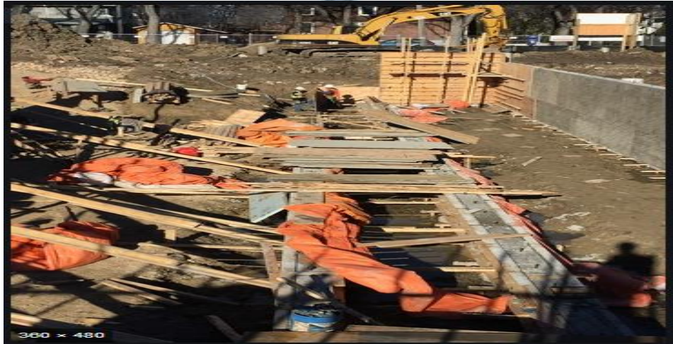
Fig 2 De-nailed formwork
