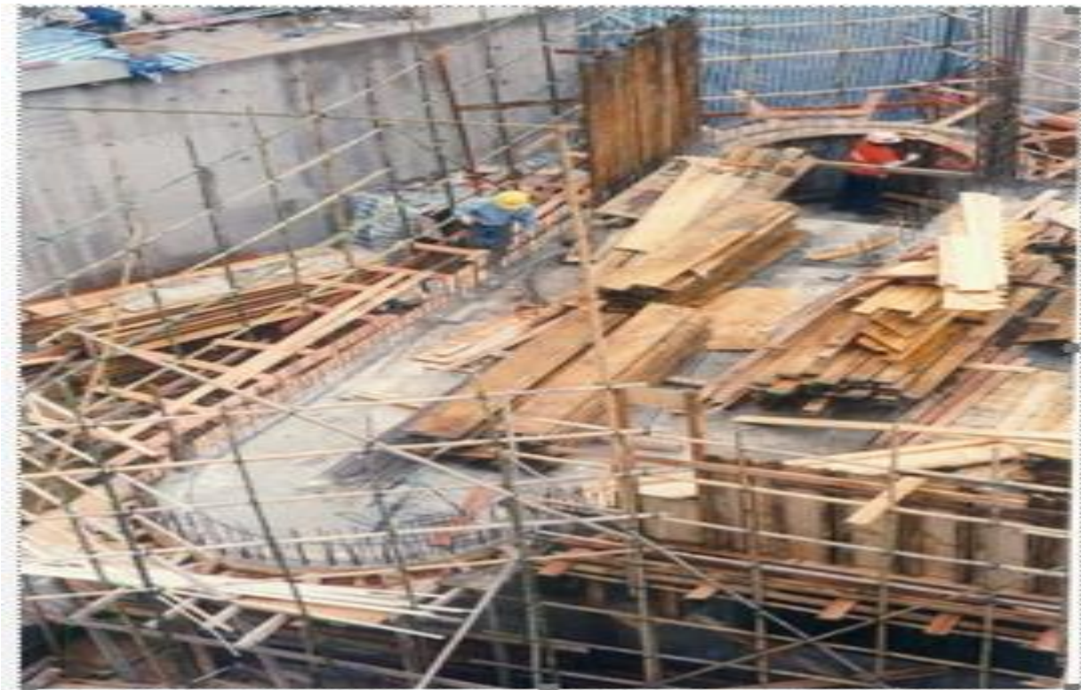
Fig 4 Stripped formwork components
